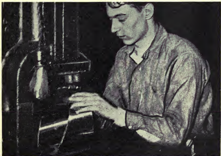
TRIMMING SHEETS AND SEWING DUCT ELBOWS
